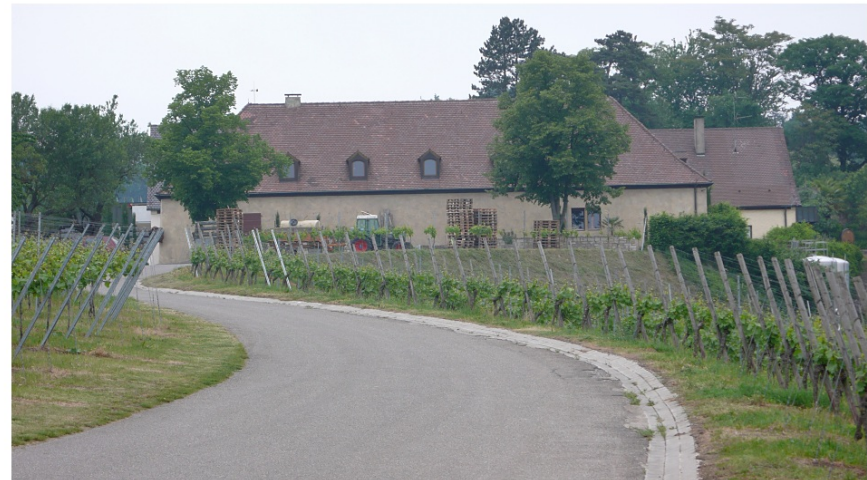
After : The exterior of the back entrance of the house on the vineyard.
